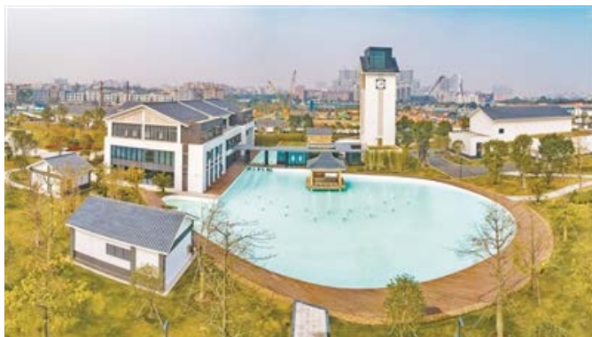
Photo of the Shijing Sewage Treatment Plant
