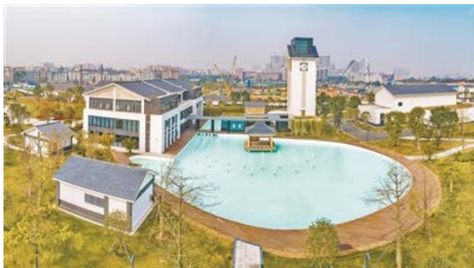
Photo of the Shijing Sewage Treatment Plant
