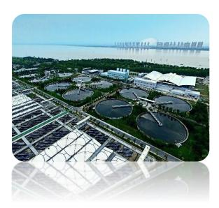
A wastewater treatment project located in the eastern China, consisting of the expansion of an urban sewage treatment plant together with the laying of supporting pipeline. So far, the project has been completed. The annual sewage treatment capacity of the project in 2018 is 16.23 million tons. The direct reduction of pollutants are as follows: COD: 1,860 tons / year, NH<sub>3</sub>-N: 90 tons / year.
