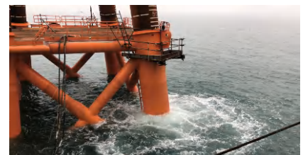
Use of bubble curtain as mitigation measure to further reduce underwater noise from piling during jetty construction
