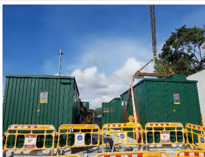
Delivery of package substations
