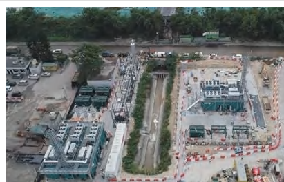
An overview of the project site
