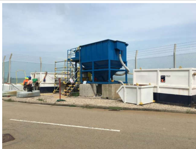
Site waste water treated with desilting and water treatment plant before discharge
