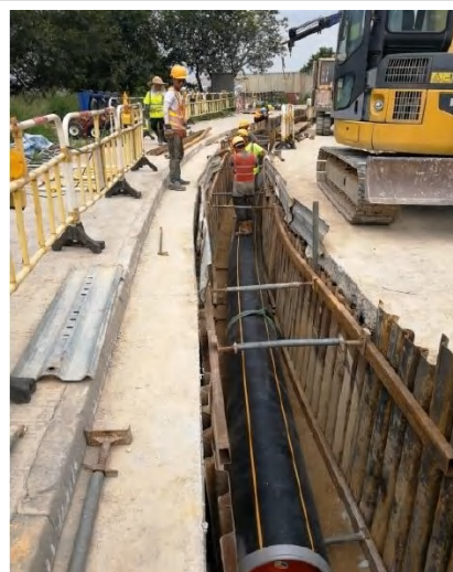
Gas pipeline laying along Nim Wan Road
